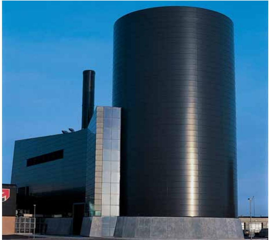
Gas fuelled combined cycle CHP plant 55 MW elec /55 MW heat with heat accumulator, owned and operated by Hjørring District Heating Company, a consumer owned cooperative.
