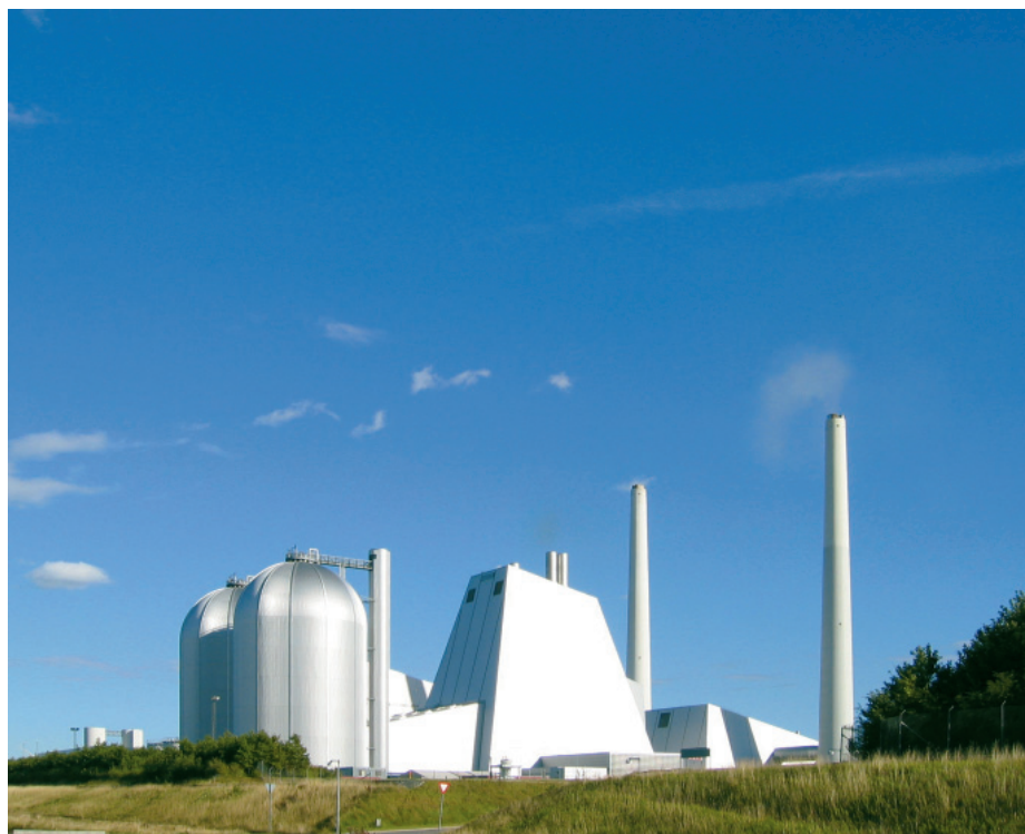
Photo 1. Heat accumulators at Avedøre Power Station.
