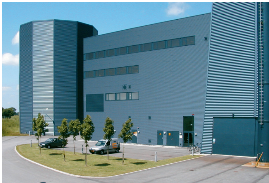
Photo 2. Heat accumulator at Maribo-Sakskøbing Local CHP Station.
