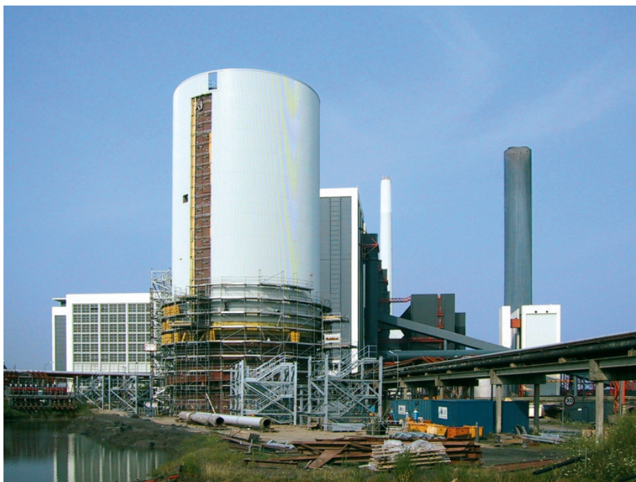
Photo 3. Heat accumulator at Asnaes Power Station under construction.
