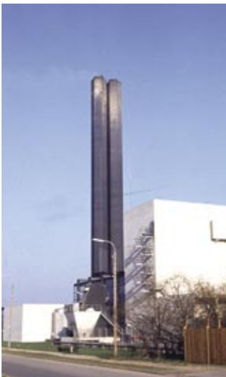
Nordforbrænding, commissioned in 1969, Architect: Finn Monies
