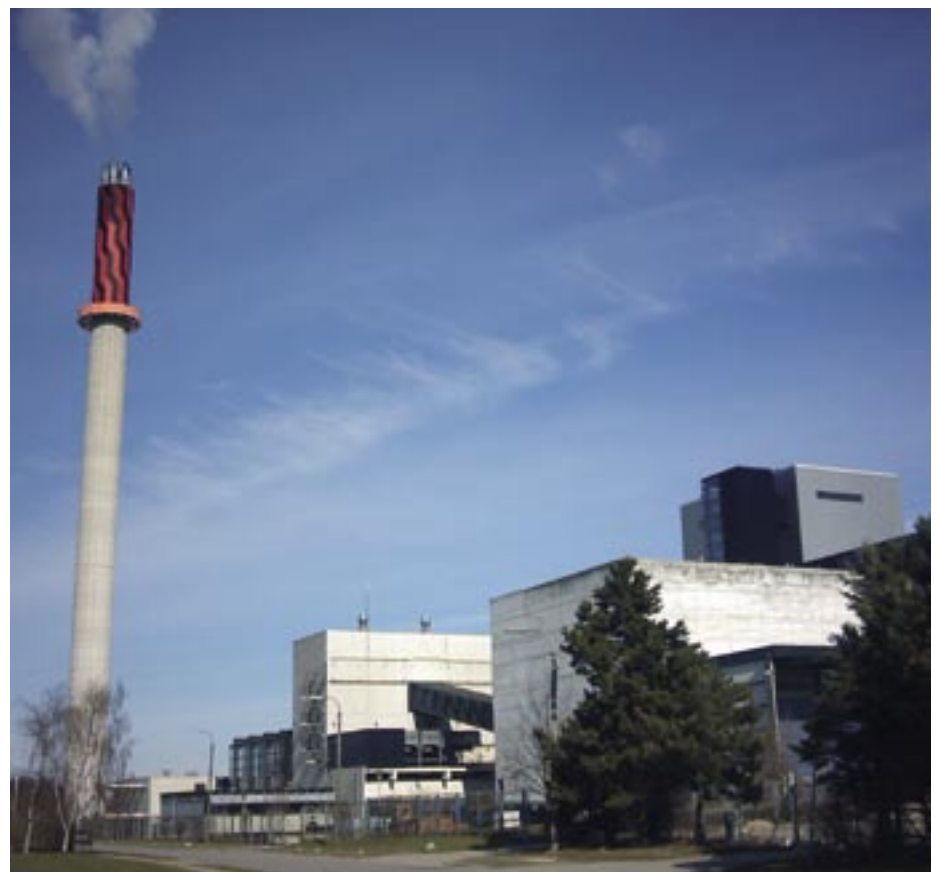
Nordforbrænding today, after it has been extended by a new CHP line. Architects: Cubo Arkitekter A/S
