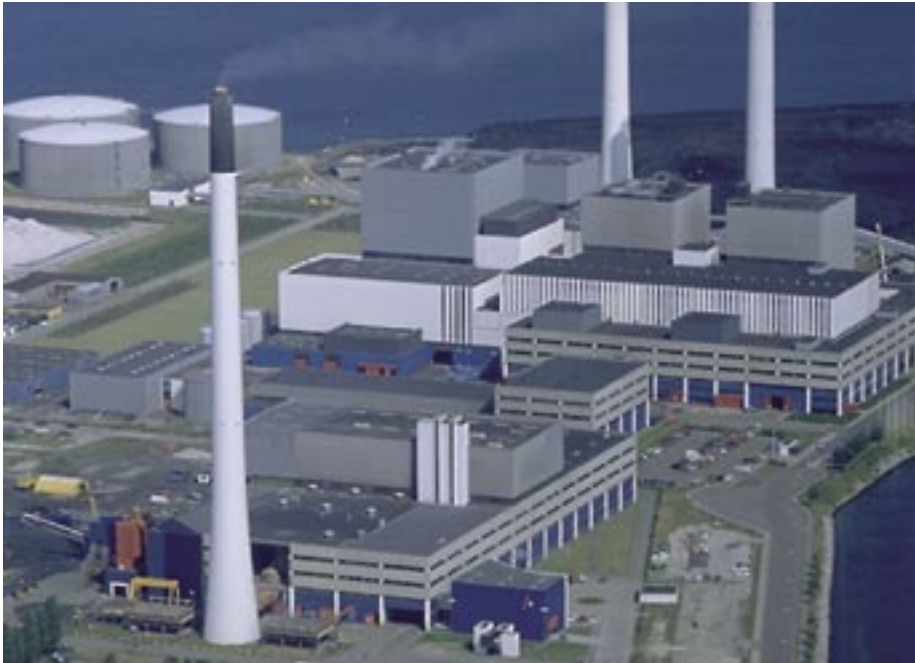
Amgerforbrænding and, in the background Amagerværket (see the following article). Both plants were commissioned in 1970. Architect: Jørgen Maglebye
