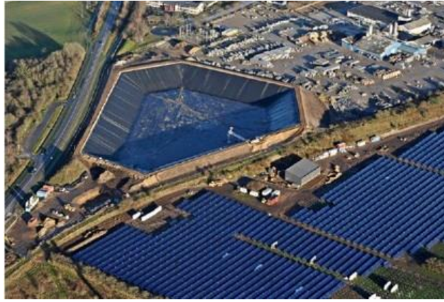
Figure 6. The Vojens pit heat store and the solar collectors
