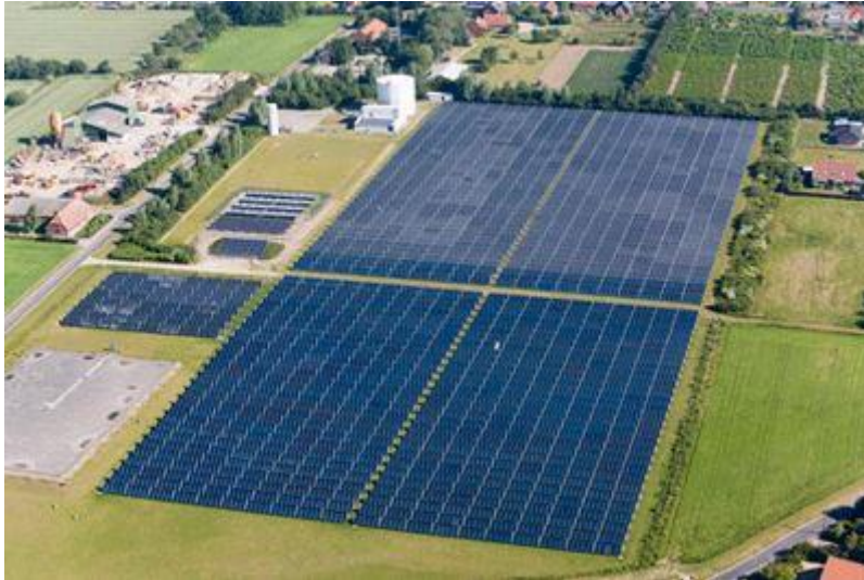
Figure 11: Marstal Fjernvarme solar collector system with heat accumulator
